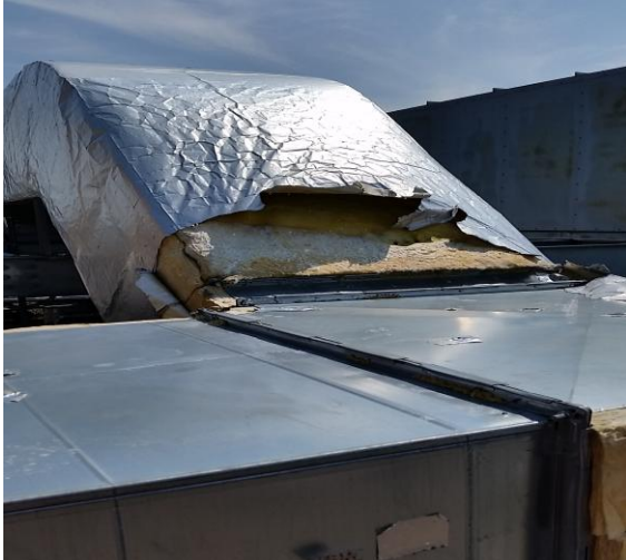
Missing and damaged air duct insulation
