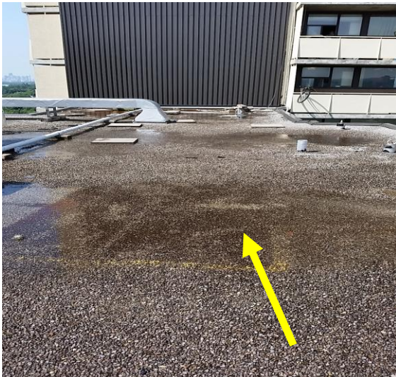
Ponding water on 35% of the roof
