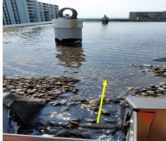
Blocked drains and creating ponding water
