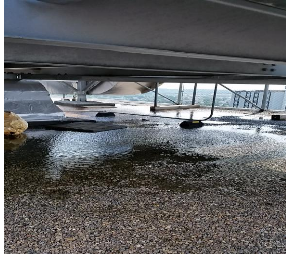
Ponding water and debris under roof top units
