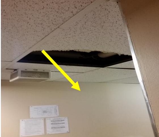
Arrow indicates a roof leak in the hallway
